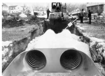
Multiple End Section on Round CSP
