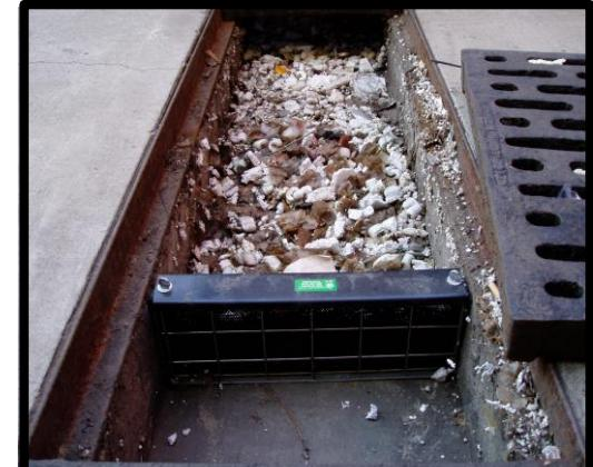
**TDAM - FOG Installed in a trench drain**
