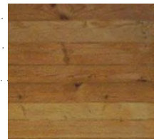
WOOD LOOK SYSTEM SOFFIT AT ENTRY
