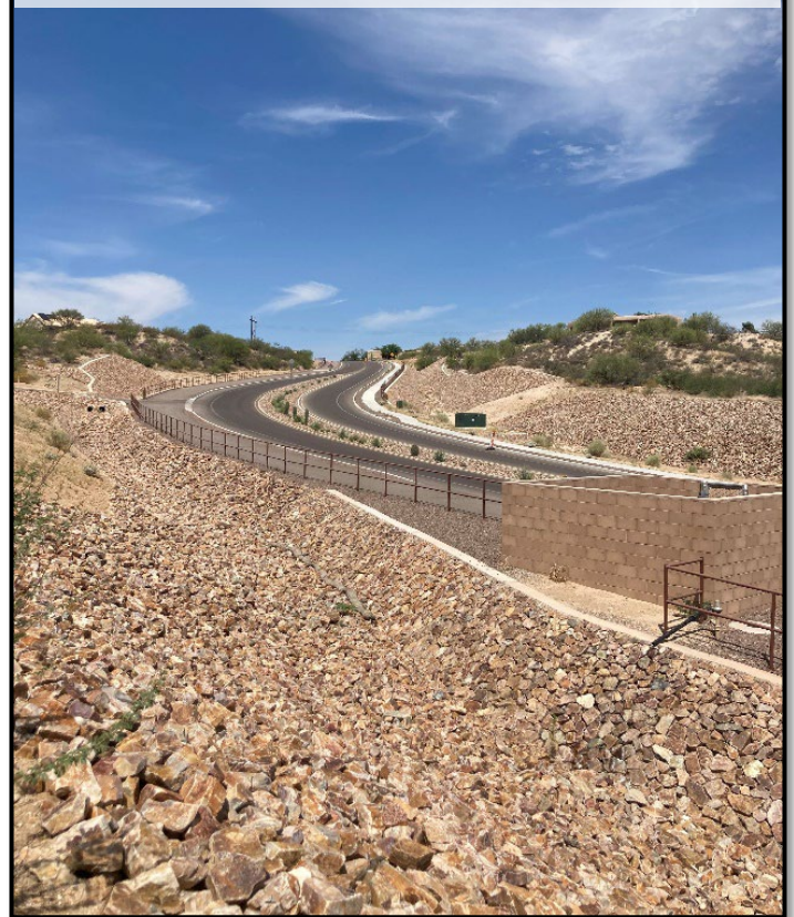
Newly Constructed Drainage Channel Along the Project's Frontage and Moore Loop
