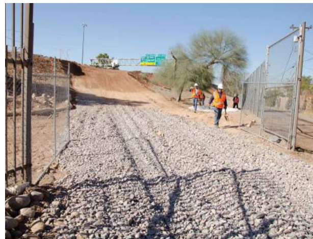
Fencing ensures vehicles enter / exit at trackout.
