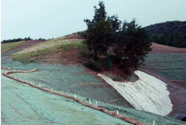
Mature trees preserved in place. Notice sediment wattles, erosion control blanket, seeding and mulch cover BMPs used in combination to achieve the most effective erosion control for these site conditions.
