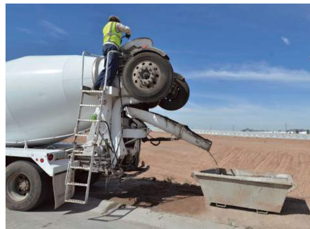
Slurry residue must be properly captured and contained.
