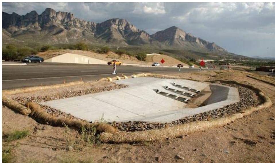
Rock mulch and sediment logs used to protect storm drain inlet.
