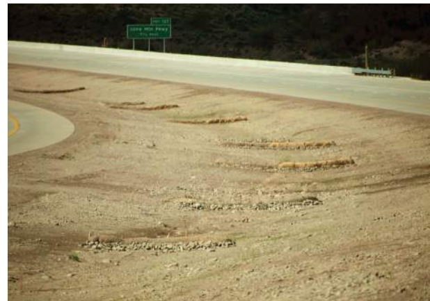
Sediment logs used as check dams.
