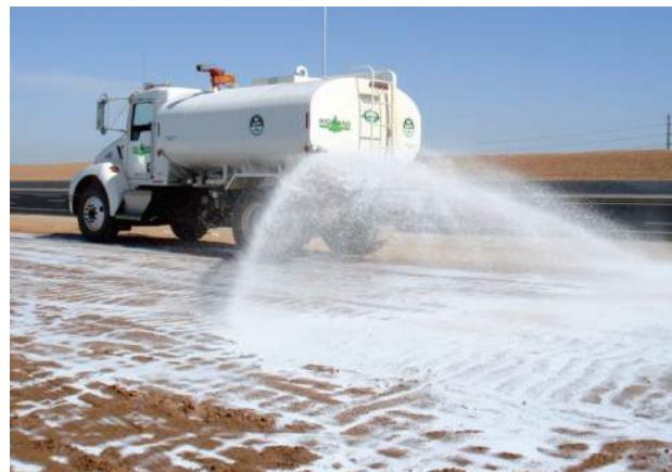
Application of soil binder.
