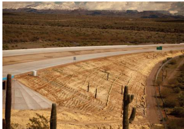
Sediment wattles spaced on a slope.
