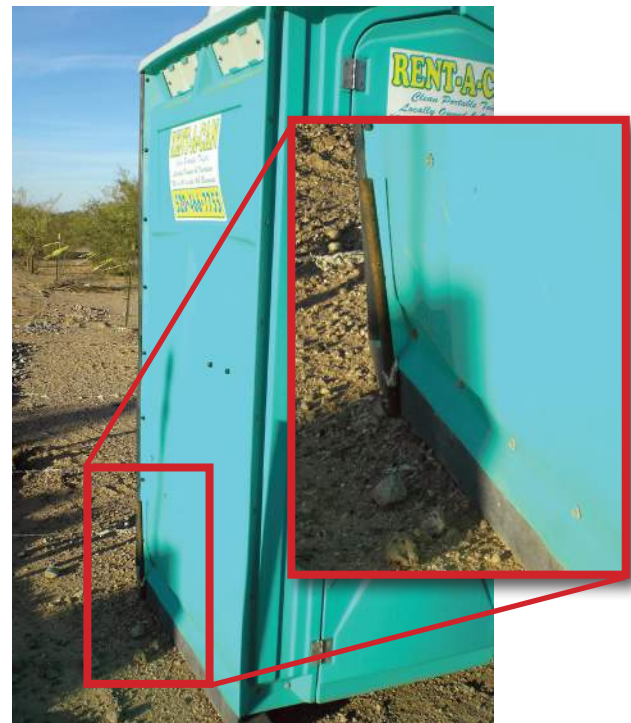
Staking is the preferred method for securing portable toilets.
