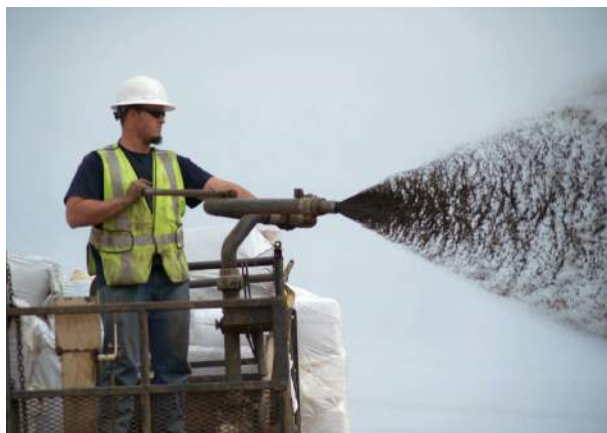
Hydraulically applied compost may be used on slopes steeper than 3:1 or where broadcast application is not feasible.
