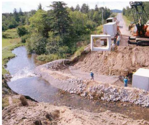
A flow bypass channel is used during placement of a multi-section culvert. Note the clear water in the diversion channel.
