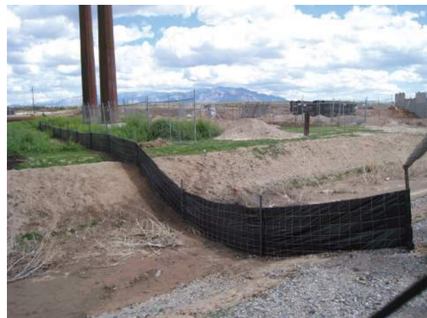
Do not use silt fence across ditches or drainage channels.
