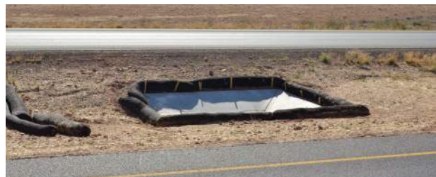
Compost socks used on slope face and as check dams (top), and as inlet protection (bottom).
