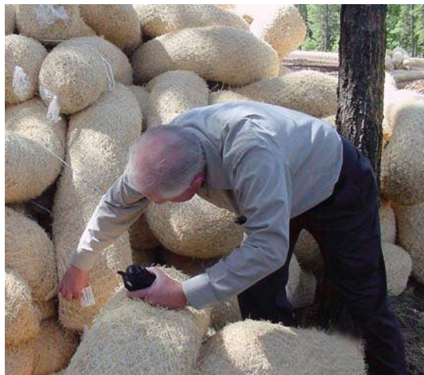
Sediment wattle inspection.
