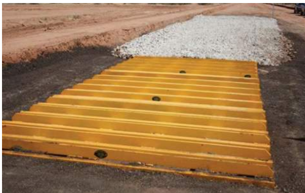
Rumble strips and gravel provide more effective track-out control than gravel alone.
