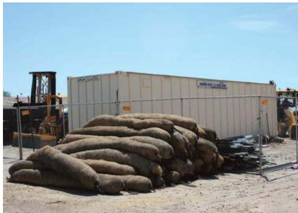
Sediment logs stored on site are immediately available for replacing damaged/displaced logs.
