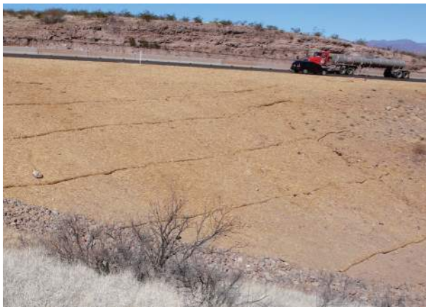
Straw mulch cover over a seeded slope.
