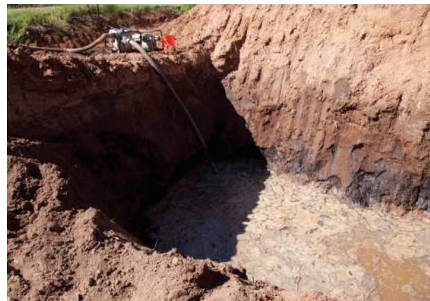
Sediment is retained in the basin during this dewatering operation.
