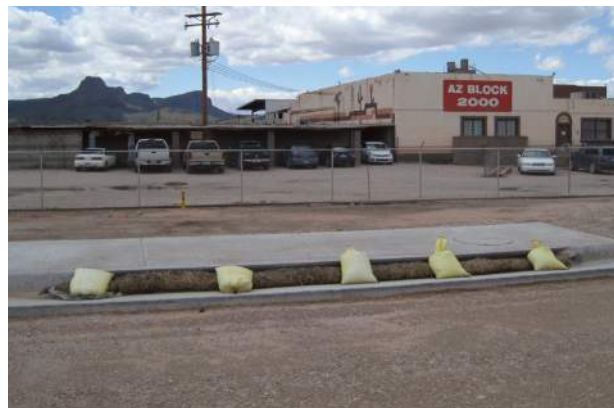
Sediment wattles held in place with gravel bags can be used to provide protection for curb inlets.
