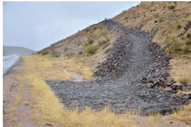
Gabion-style crown ditch used for extreme drainage conditions.
