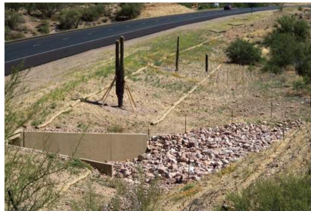
Proper sizing of rock riprap is essential to design effectiveness.
