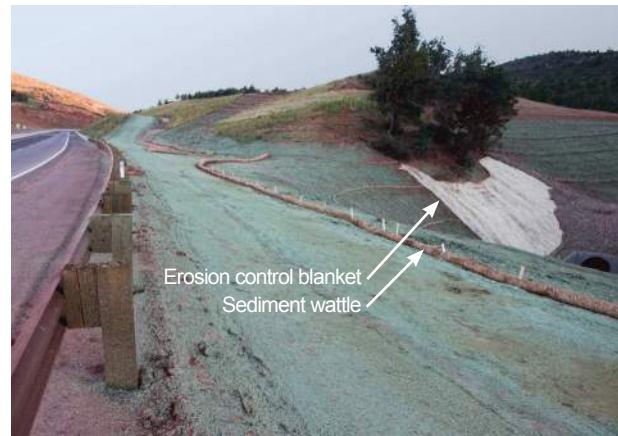
Mulch cover used in combination with sediment wattles, erosion control blankets and vegetation preserved in place.
