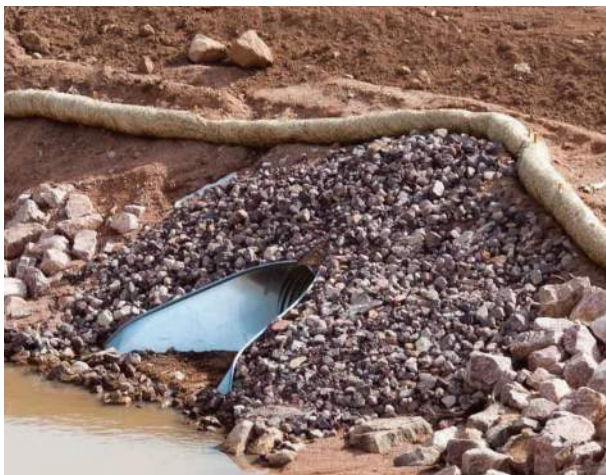
Rock at interface of soil and drainage pipe.
