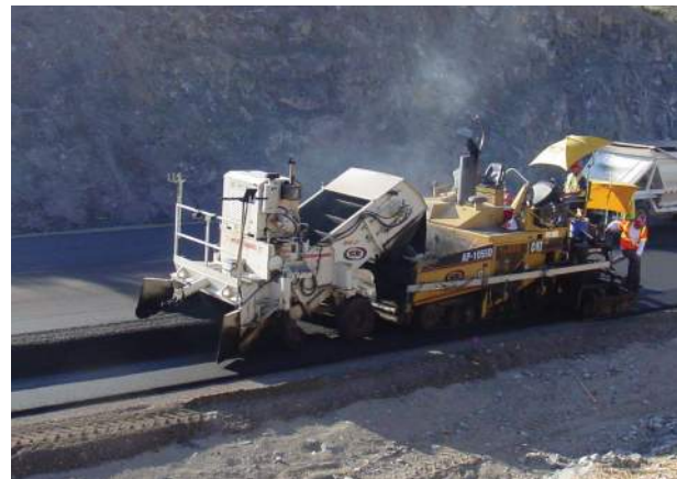
Asphalt paving operation.
