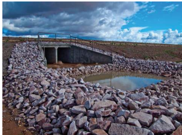
Sediment trap with rock protection.
