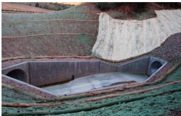
Blanket used in combination with mulch cover, sediment wattles and rock mulch.
