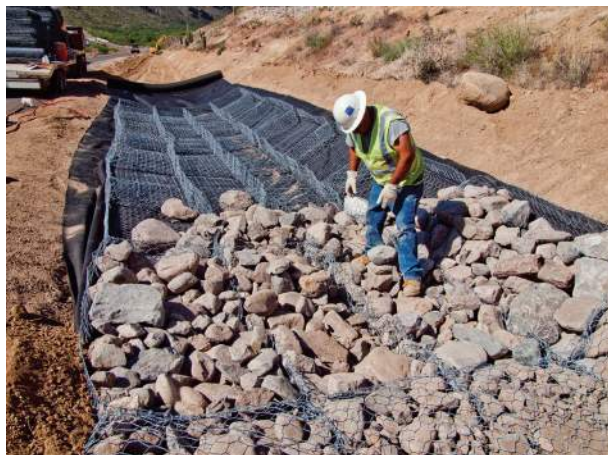
Gabion mattress designed for anticipated high-velocity flows.
