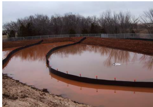
Soil may not be providing adequate infiltration.
