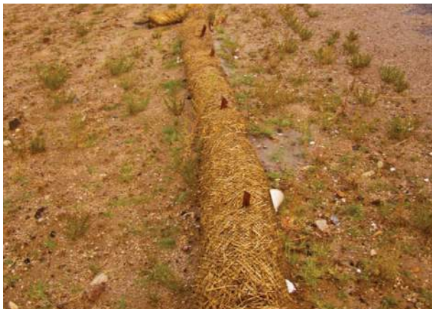
Proper staking of wattles.
