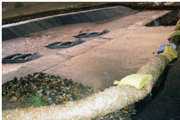
Gravel bags used to anchor sediment wattle.
