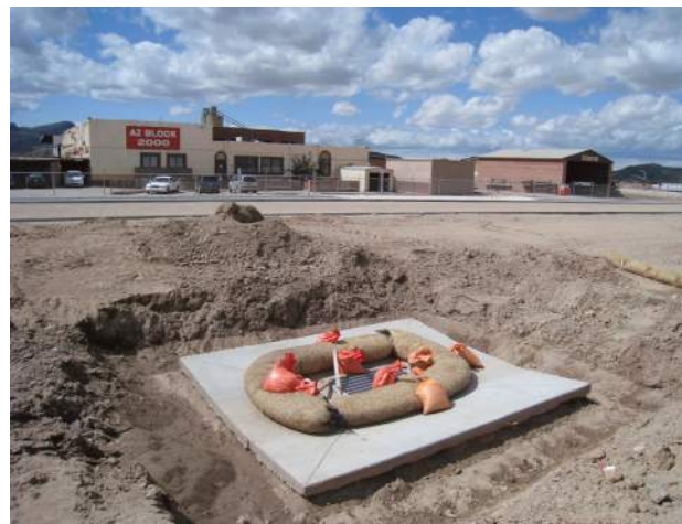
Excavation prior to rock placement at drainage structure (use gravel bags to anchor logs/wattles).
