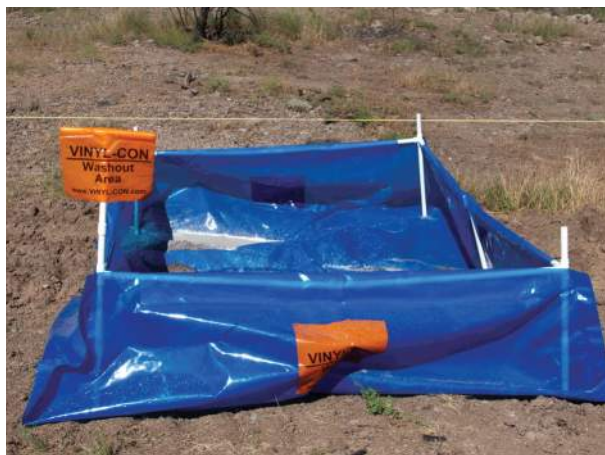
This simple containment system is appropriate for small jobs.
