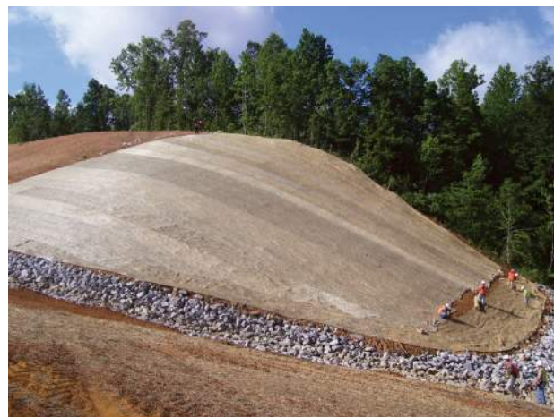
Erosion control blanket installation.
