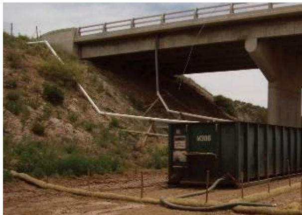
Dewatering during bridge work.
