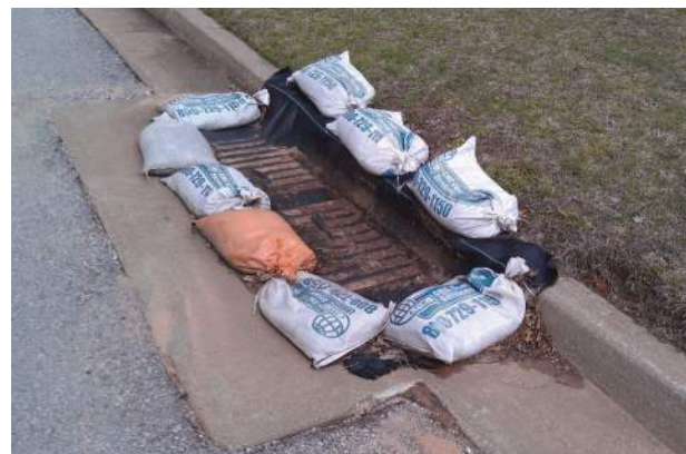
This inlet protection device is doing a good job of capturing fine sediment. Proper maintenance will help ensure continued performance.
