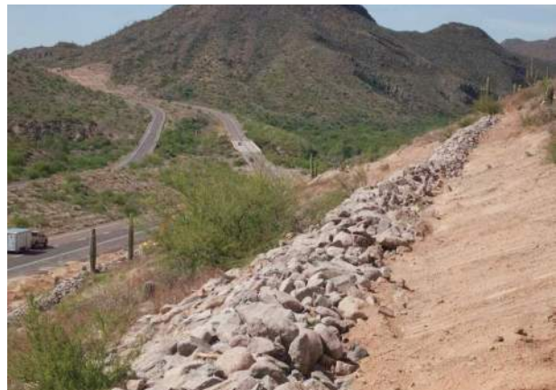
Berms run parallel to slope contours and are trenched into slope face.
