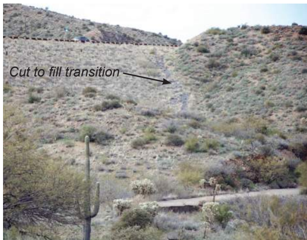
Cut to fill transition leads to stable drainage.
