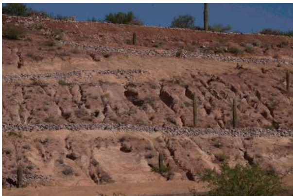
Rock berms used as a corrective measure on an eroded slope. Due to vegetation establishment, areas with rilling were not regraded.
