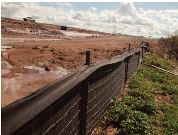
Proper wire mesh support for fabric.
