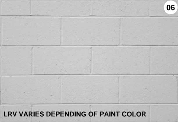
CONCRETE MASONRY UNIT: RUNNING BOND PAINTED SEE ELEVATIONS
