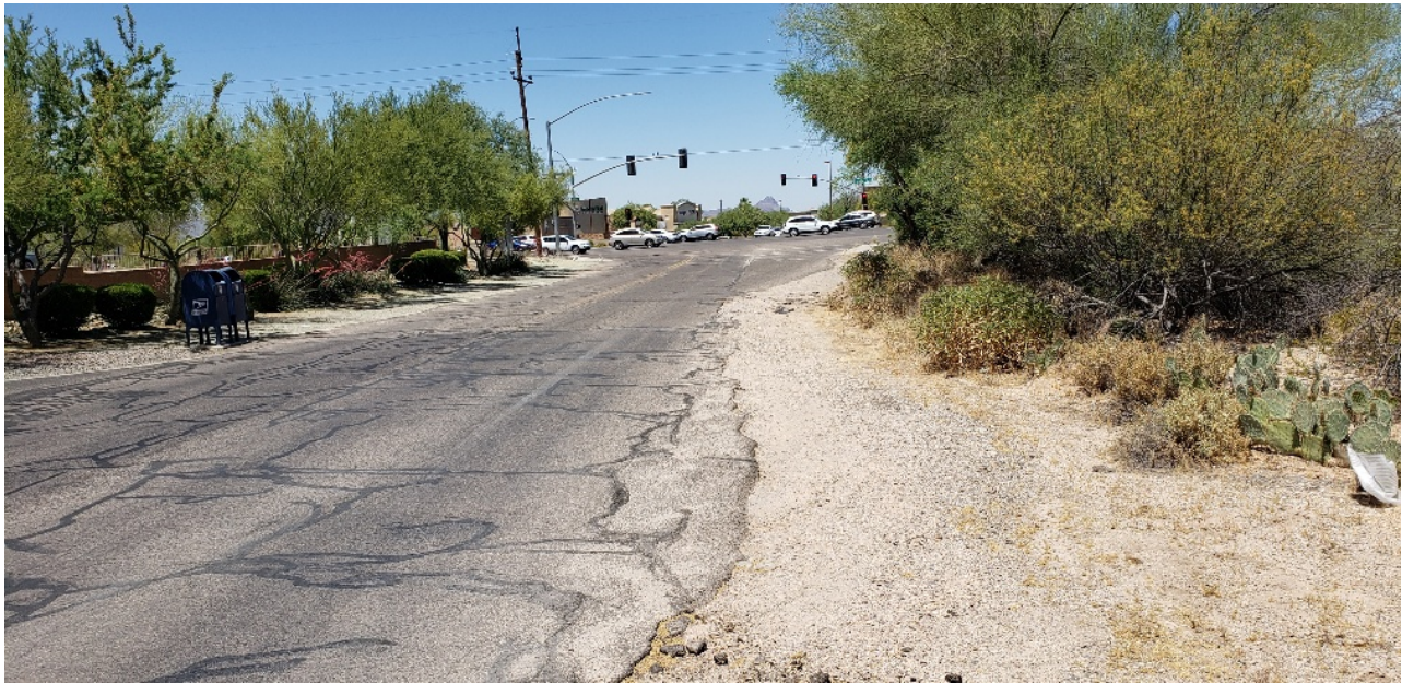
Looking West on Suffolk Drive toward SR 77 – Project Location to the Right
