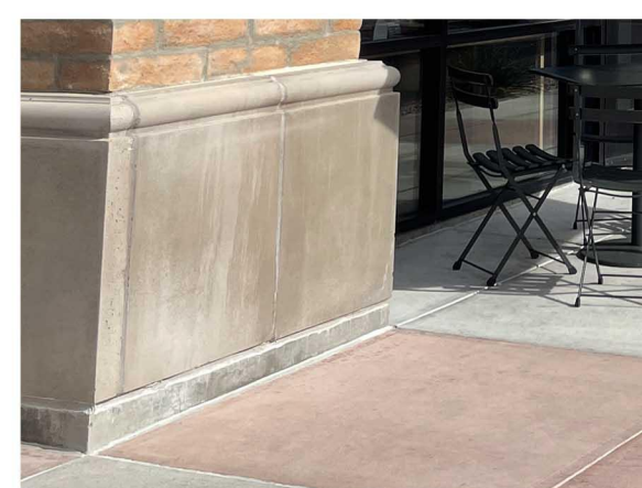
PRECAST BASE & COLORED CONCRETE SIDEWALK ACCENT
