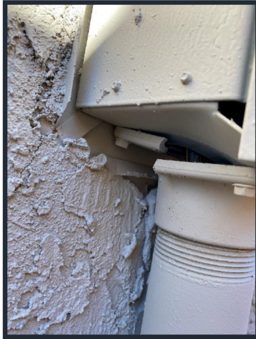
Figure 5: Lot 19, outside utility piping has separated from the base of electric box on the east side of house
