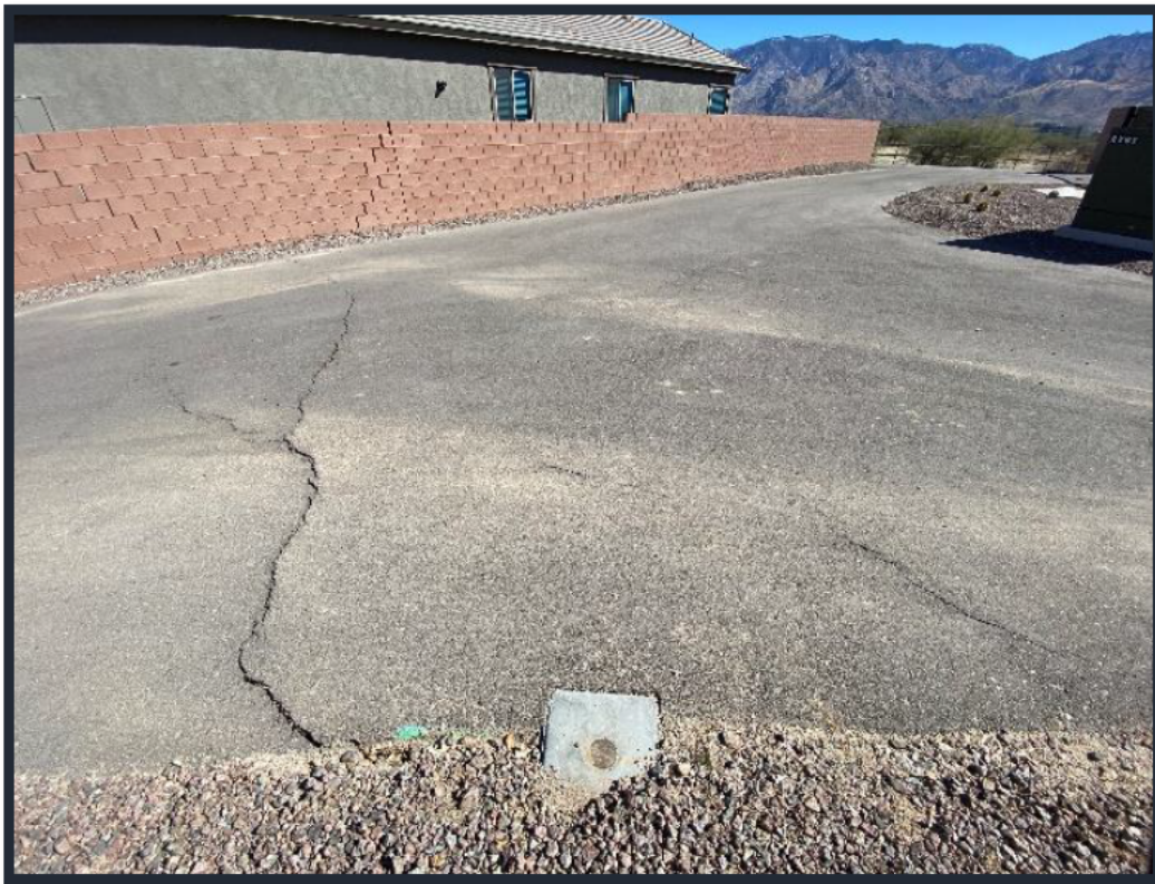
Figure 1: Cracking in common area of booster station, in the asphalt pavement, and leading to Lot 20. Similar residual cracking patterns in both wall and asphalt pavement
