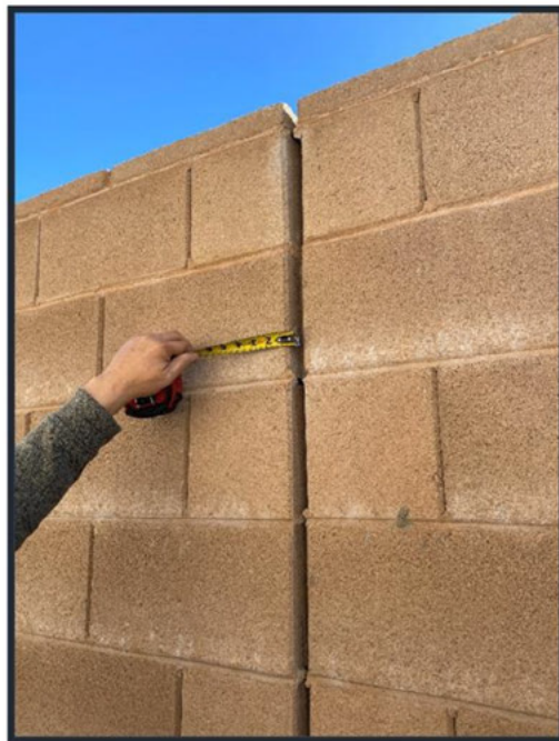
Figure 3: Lot 19 displacement and westward deflection observed in the east wall
