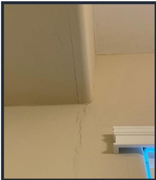
Figure 1: Lot 19 Cracks in the front bathroom, above the shower stall
