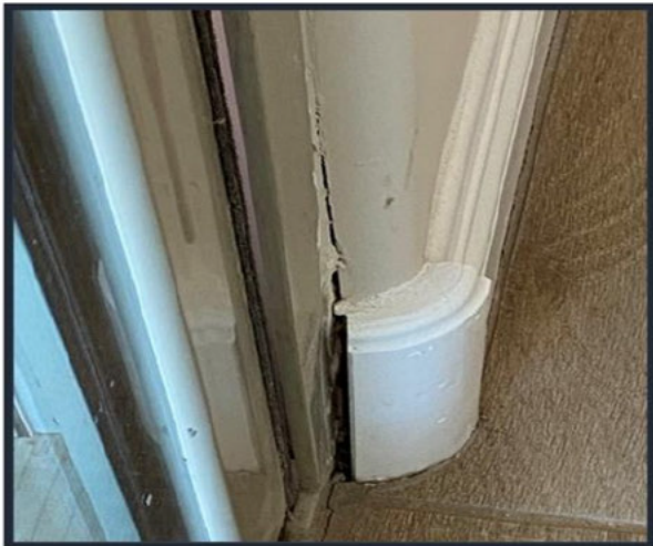
Figure 3: Lot 19 Separation of baseboard from wall, near the sliding glass door, in the dining nook
