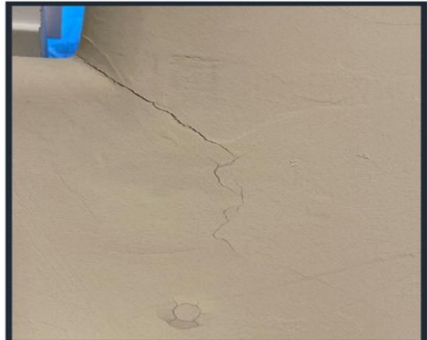
Figure 4: Lot 19 Cracks and pop-outs observed in the front bedroom
