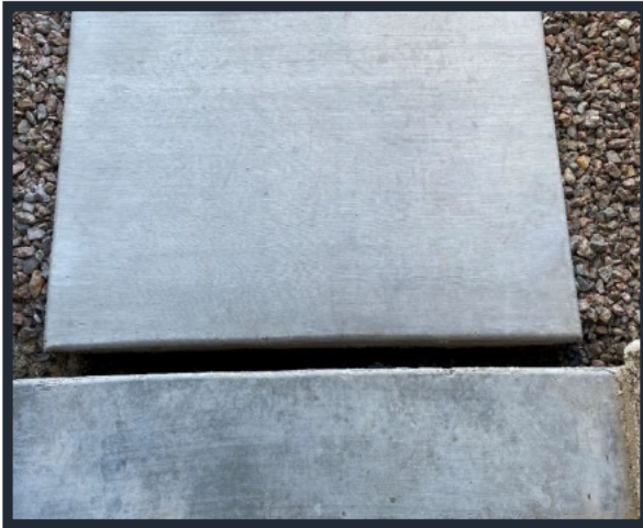
Figure 1: Lot 19, separation of concrete walkway at the front entrance of the existing house
