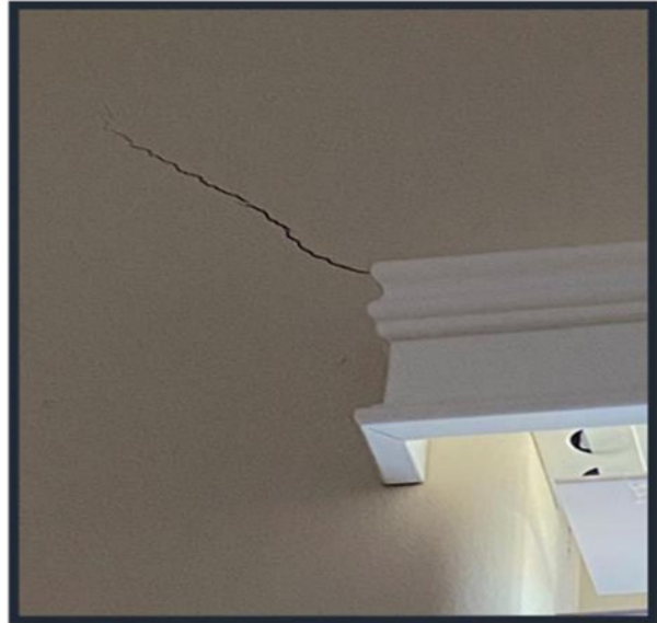
Figure 6: Lot 19 Cracks in the drywall at top edge of the window in Bedroom 2
