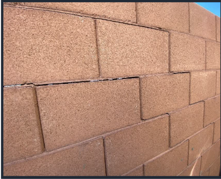
Figure 1: Lot 19 Stair-step separation of individual blocks in the wall
