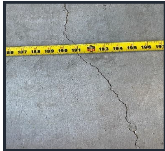
Figure 2: Lot 19, crack in the concrete slab in the garage
