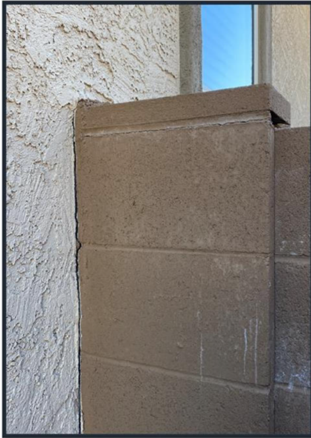
Figure 1: Separation of west block wall from residential structure
