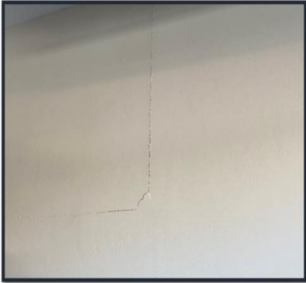
Figure 5: Lot 19, cracks in the drywall in the garage
