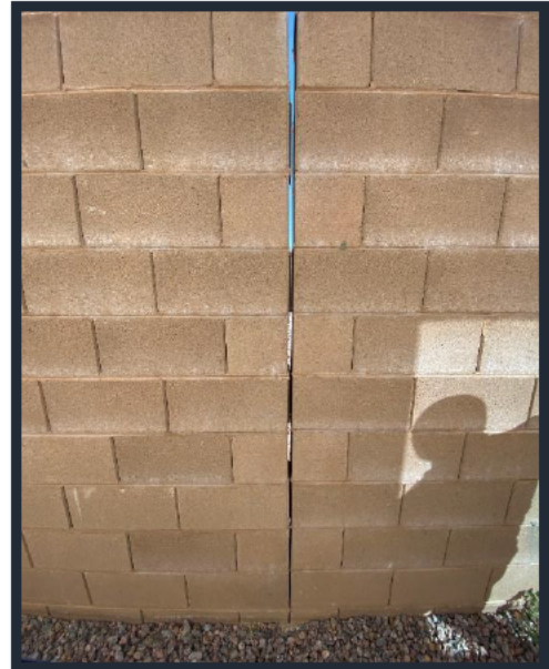
Figure 2: Lot 19 vertical separation of block wall panels
