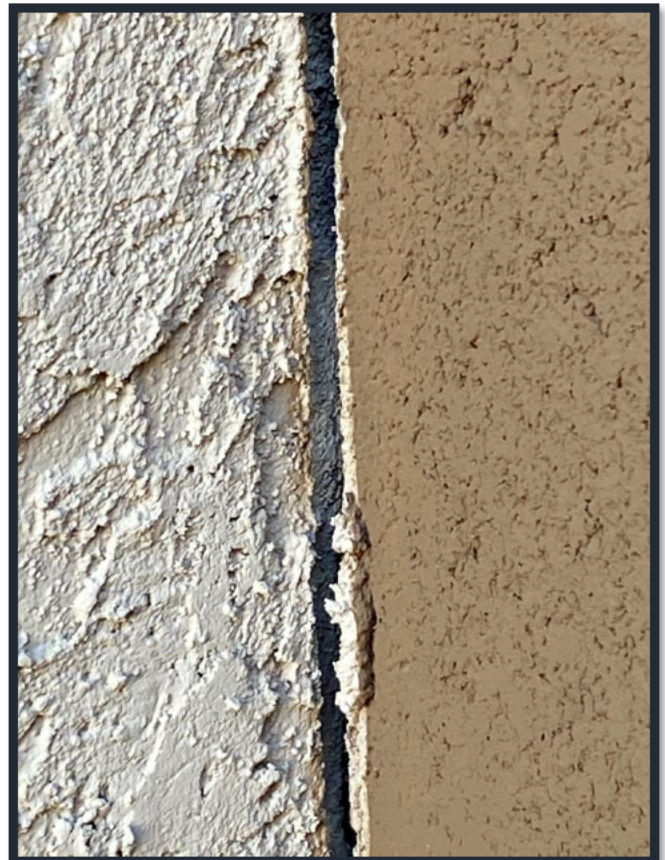
Figure 2: Close-up of separation crack on west side of house
