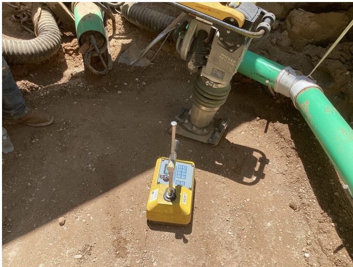
Compaction done with jumping jack.
