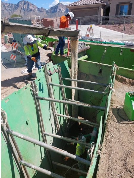
Slurry placement on the sewer line inlet repair
